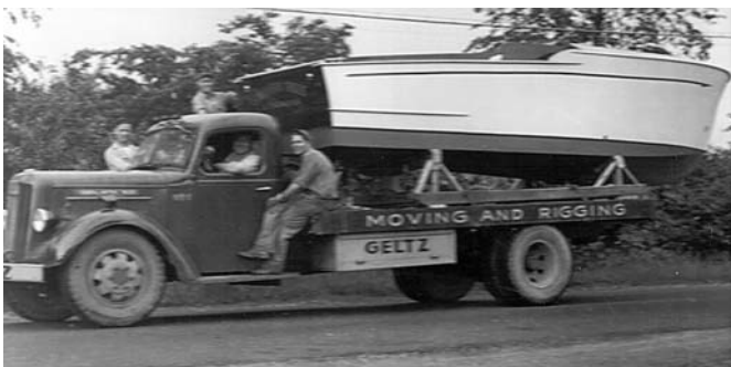
SOUTHERN CROSS moving to 867 Sweeney Street for finish work
